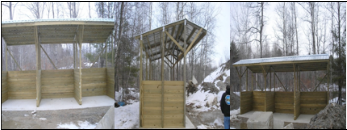
Figure 8: University of New England’s three-bin compost facility. At UNE, this 30’ x10’ (roughly 10 meters by 3 meters) ‘three bin compost facility’ has kept up with the composting needs of the animal remains generated at UNE Marine Animal Rehabilitation Center for the past 5 years. In that time, approximately 38 piles of marine animal soft tissue have been composted (approx. 15 tons).
